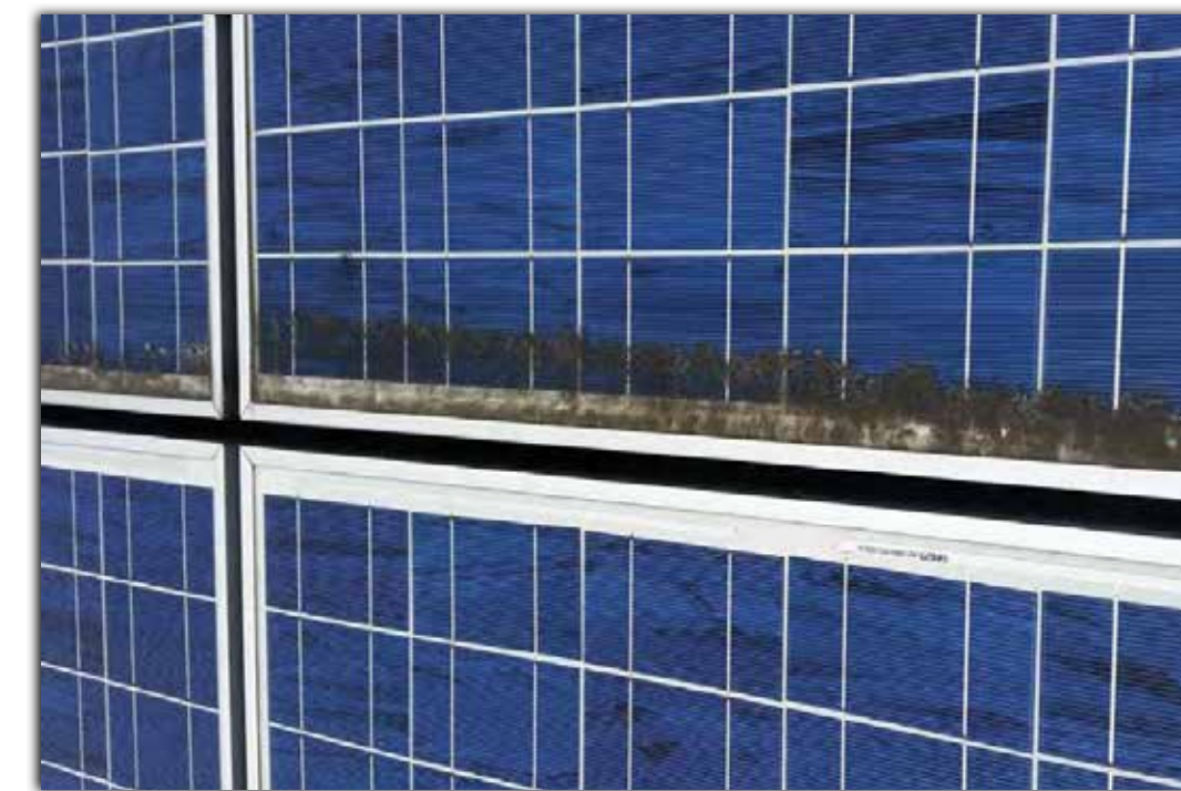
Dirt, dust and shading lead to Hot-Spots
